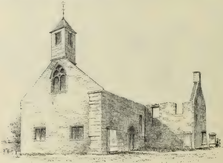
FIG. 1600.—Stow Church. View from South-West.
